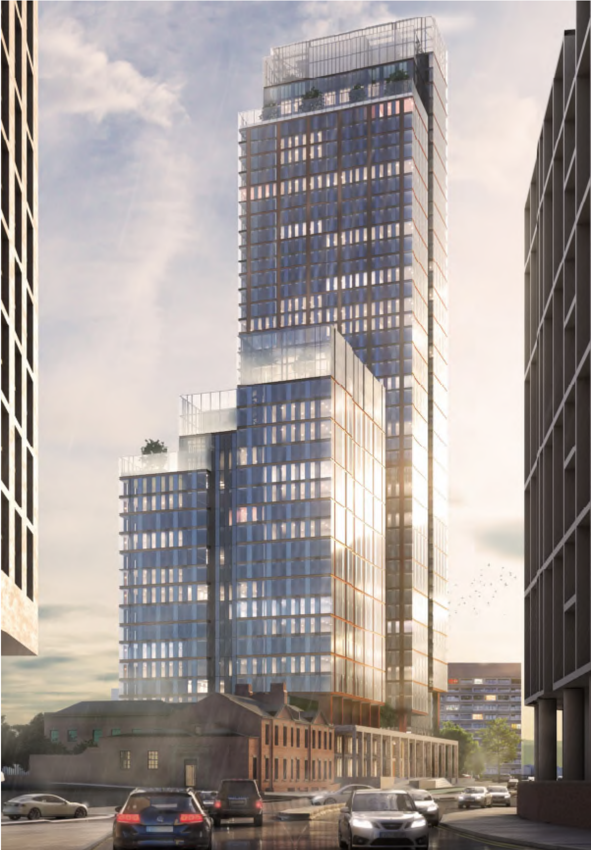
View looking south west along Chester Road
